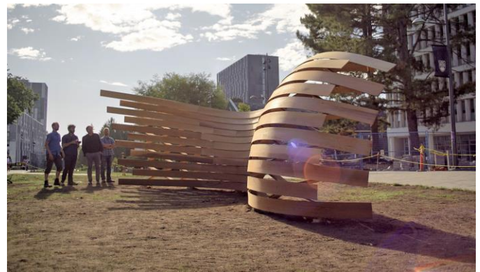
2017 - Robot Made Workshop prototype: Double-Layered Diagrid Facade Structure
