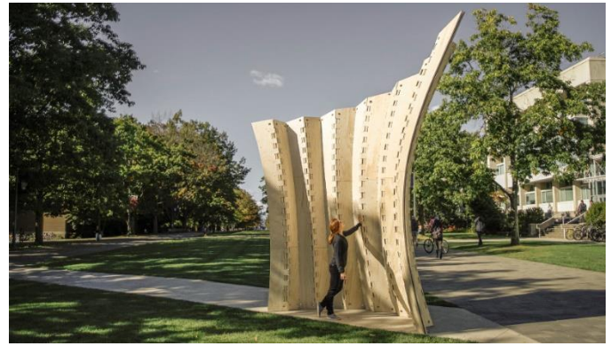
2016 - Robot Made Workshop prototype: Double-Layered Elastic Bending for Large Scale Folded Plate Structures
